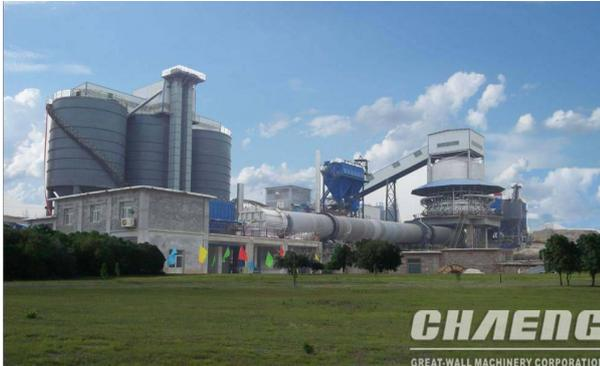
Lime production line is a complete production line that includes vertical preheater, rotary kiln, grate cooler, raw material conveyor system, finished product conveyor system, air treatment system, raw coal grinding system, and so on.
